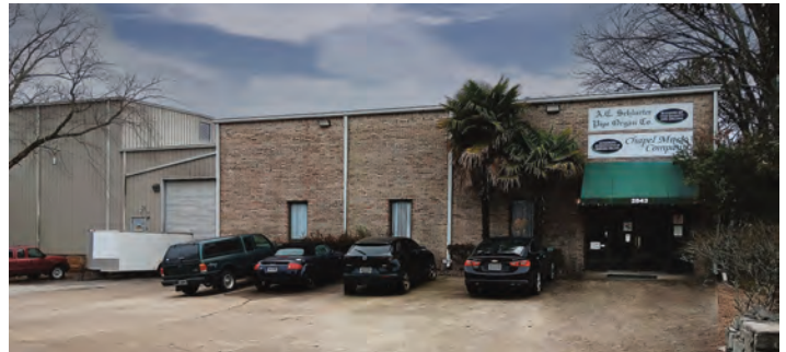
Schlueter office and shop building
