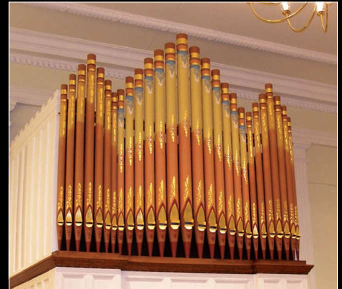
First United Methodist Church Restored facade and pipe organ repairs in Wetumpka, Alabama
