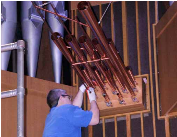
Marc Conley reinstalling the 8' Tuba Mirabilis after revoicing and modification to the supporting racks. (Photo credit: Brian Oliver)
