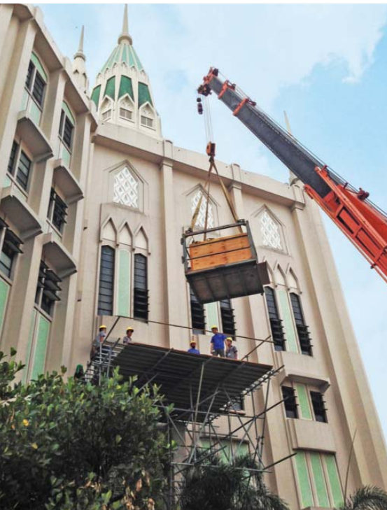
Hoisting console into building (photo credit: A. E. Schlueter III)
