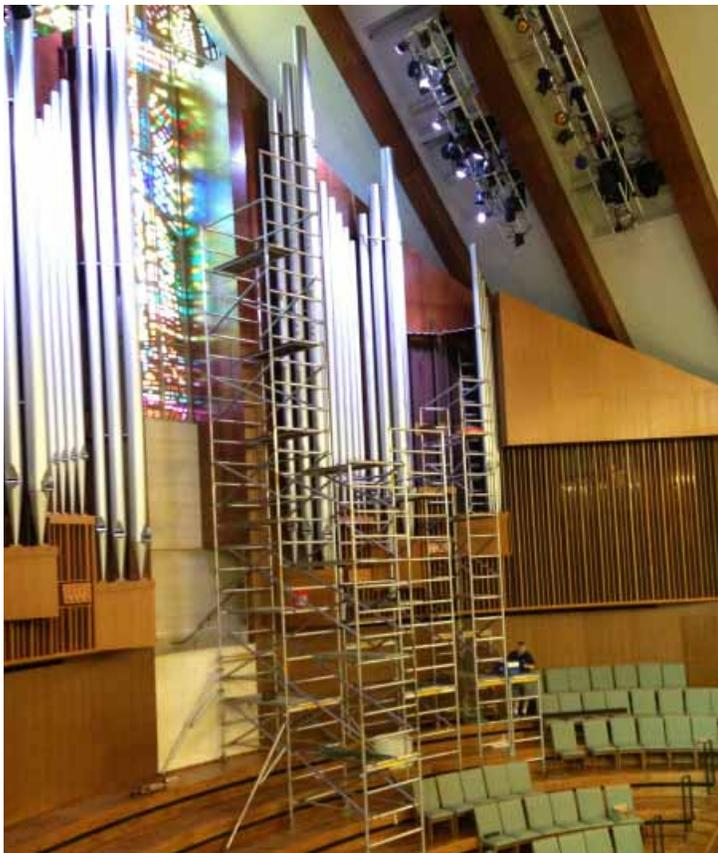
The organ facade pipe racking and structure had to be rebuilt with a significant amount of lumber and steel. Seen here is some of the scaffolding used to work on the 32' Violone pipes. (Photo credit: Brian Oliver)
