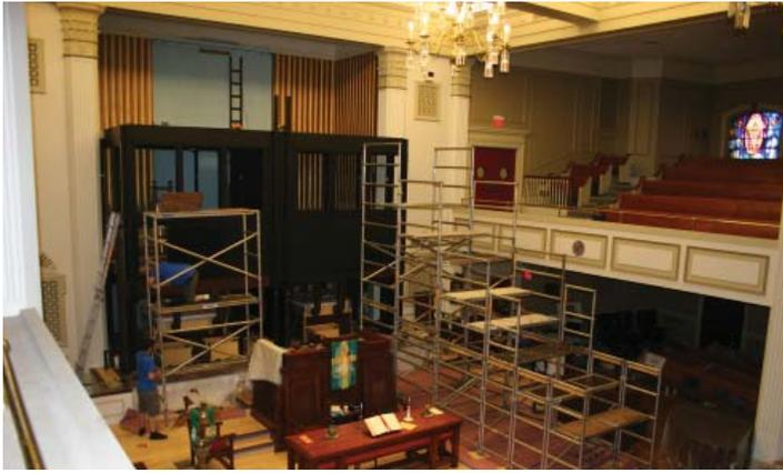
Scaffolding is erected for hoisting windchests and reservoirs to the Great and Pedal divisions on the upper level (photo credit: Jim Wilmer)
