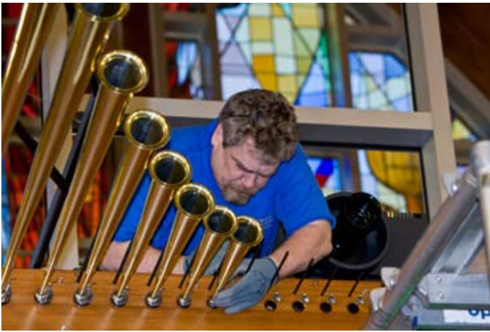
Marc Conley installing Trompette En Chamade in Antiphonal organ
